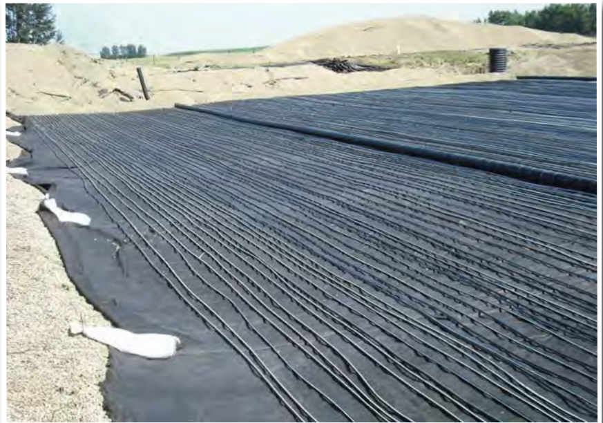
As over 758 litres of propylene glycol can be used for deicing a plane, BOD requirements become very high.
