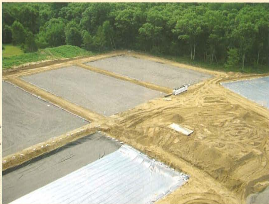
Pilot-scale testing determined that engineered wetlands currently under design for Buffalo Niagara International Airport could remove 96 percent to 97 percent of target pollutants from deicing operations.
