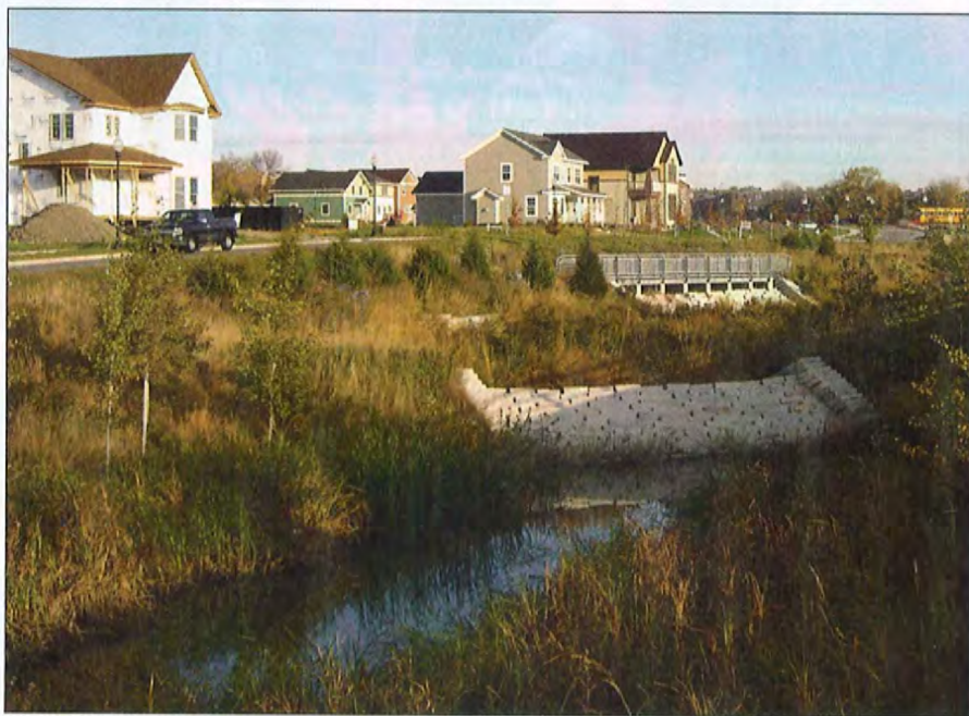
A stormwater control system retards flow and allows infiltration at the Heritage Park Development in Minneapolis.
