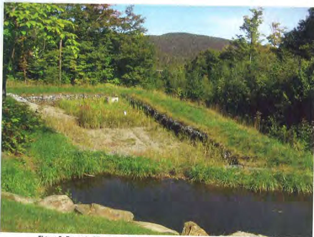
Figure 3: Example SF constructed wetland with integrated water-quality treatment
