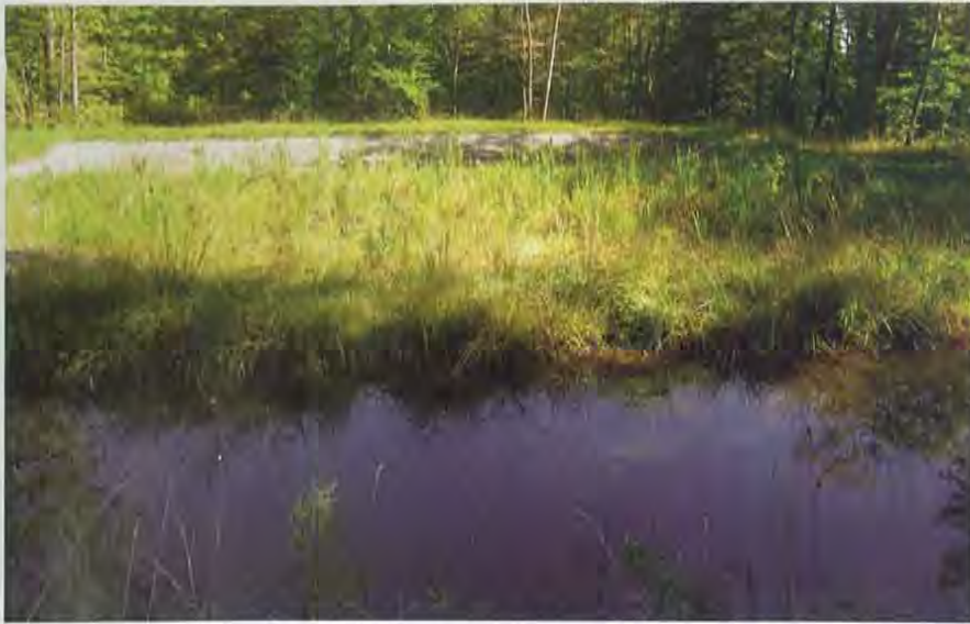
Figure 4: Typical constructed wetland at Jay Peak. The sediment forebay is shown in the foreground, followed by the SF constructed wetland and dry detention pond.
