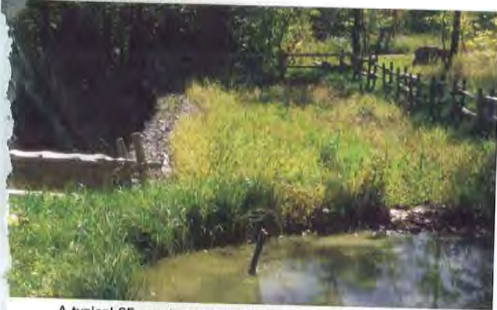
A typical SF constructed wetland configuration at Jay Peak
