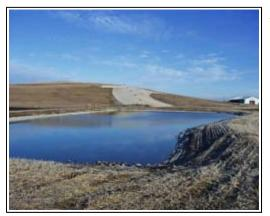
Photo: The wetland system at the Anoka County landfill exploits natural processes to remove metals from the leachate.
