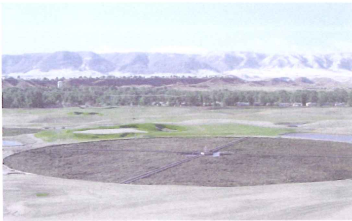
Engineered wetlands provide treatment for chlorinated hydrocarbons at a British Petroleum remediation site in Casper, Wyoming. Photo by Naturally Wallace Consulting
