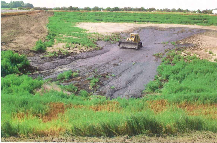
To improve reuse water quality at their facilities, Christensen Farms constructs wetlands for tertiary treatment of wastewater at this Norfolk, MN, hog farm.
