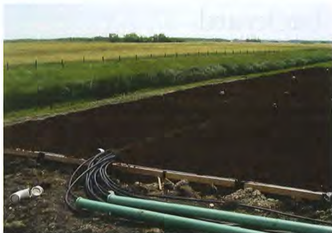
Steinbach SAGR Under Construction
