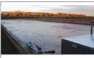
Full scale demonstration of wetland aeration for treatment of deicing fluid from Heathrow Airport in London
