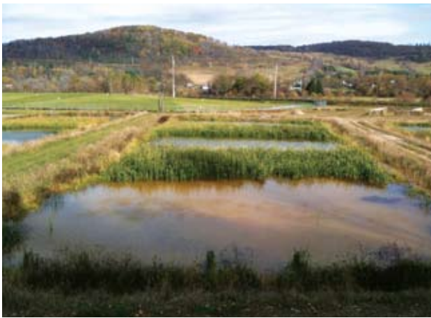
Surface flow wetland for aniline and nitrobenzene removal in Wellsville, N.Y.
