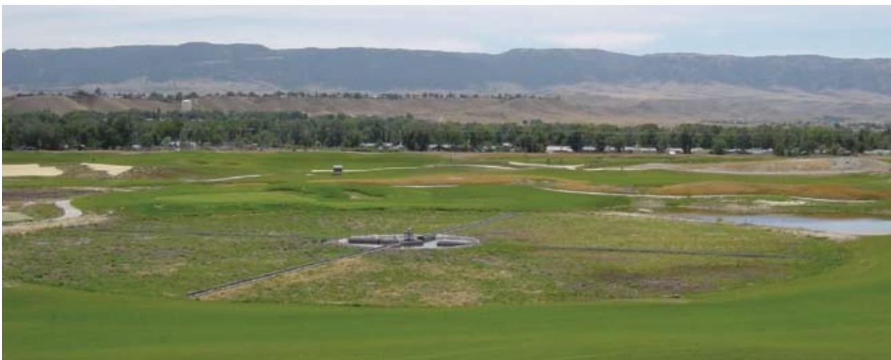
Engineered wetland for benzene removal in Casper, Wyo.
