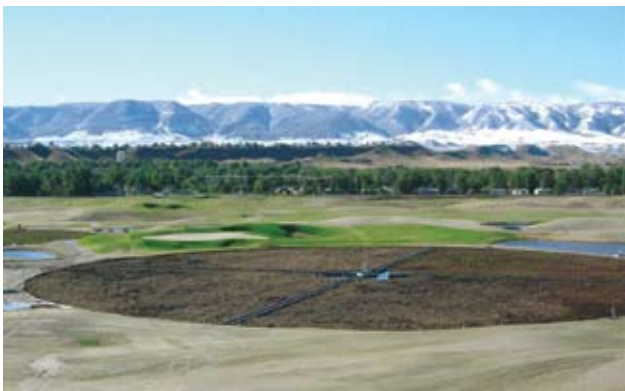
Engineered wetland under construction in Casper, Wyo.
